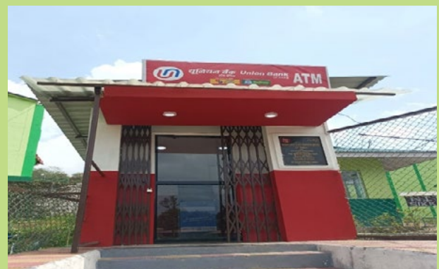
Fig.3 Single Unit Room for ATM facility
