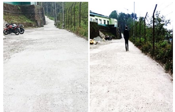
Fig.5: Repair of Road by using Cement concrete
